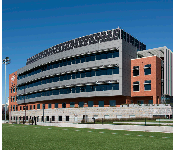
AlexRenew Environmental Center © Eric Taylor Photography
