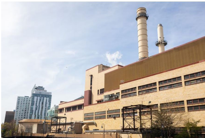
The Kendall power plant in East Cambridge is being re-fitted to generate steam power by drawing water from the Charles River. NATHAN KLIMA FOR THE BOSTON GLOBE
