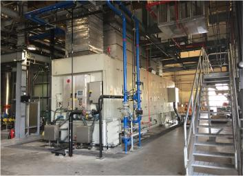
This project, a \$127 million, 42 MW new and innovative style CHP, uses cleaned digester gas produced at the plant mixed with natural gas to provide renewable energy using turbine engines and HRSGs as the prime movers.
